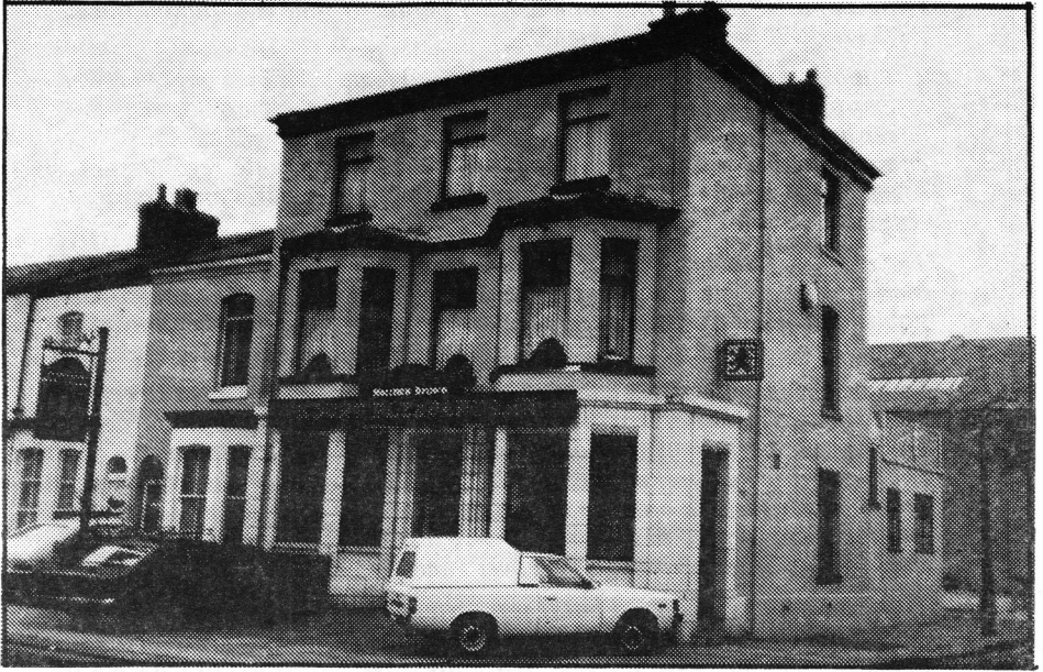
Mount Pleasant, North Shore, Blackpool – a Good Beer Guide listed Matthew Brown House.
